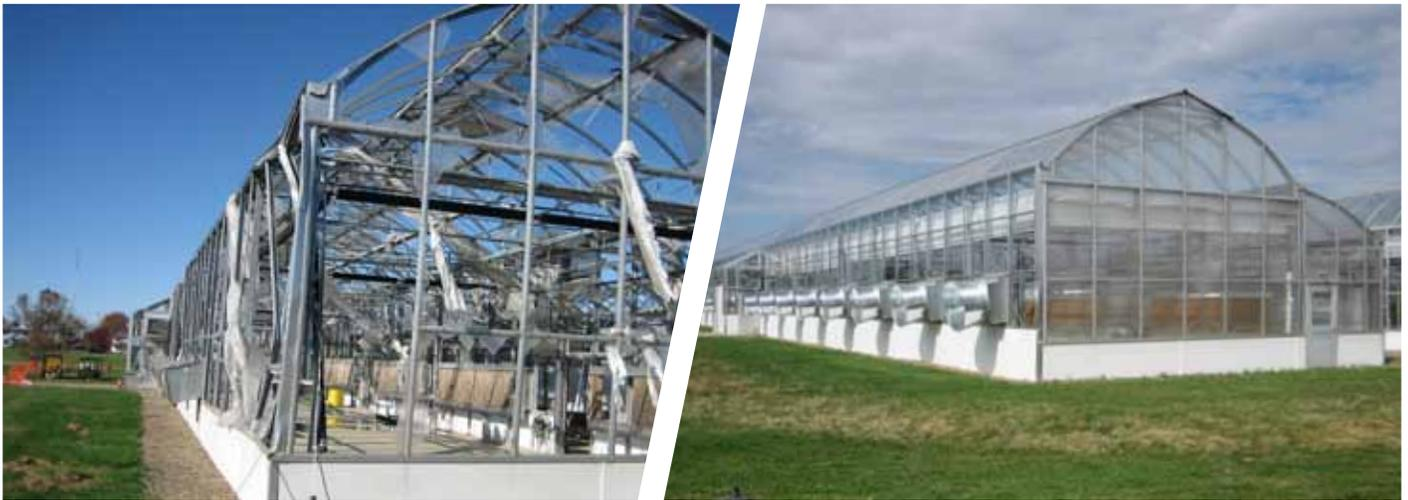
Gourley Greenhouse, OARDC Wooster, Ohio after tornado damage, and the repaired structure with new curved glass roof.
