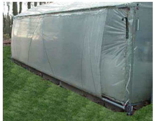
FIGURE 2 ROLLUP CURTAIN IN LOCKED DOWN POSITION WITH AIR INFLATION
